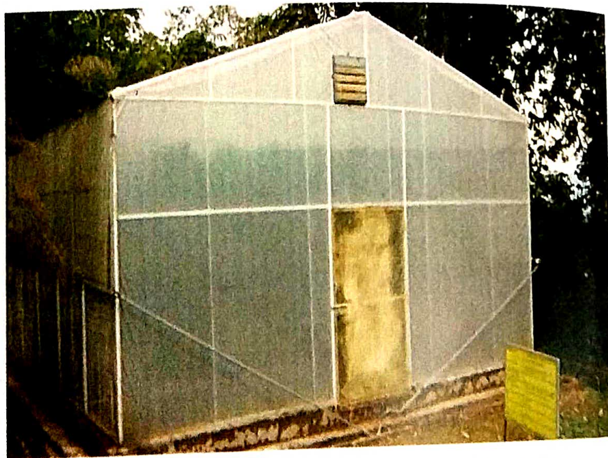
Design of the polyhouse constructed at five different locations of Sikkim for secondary hardening of tissue cultured plants
